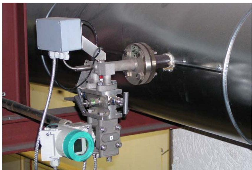
Steam flow metering with direct installed transmitter and integrated directly temperature measurement
